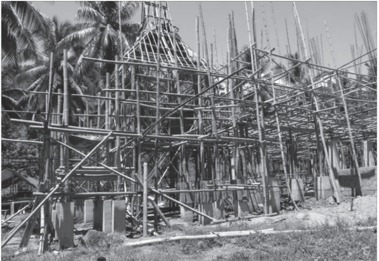
FIGURE 10.1 • The strength of a bamboo structure is best analyzed as frame—or a network of connections—rather than focusing on a connection of a member to the other
